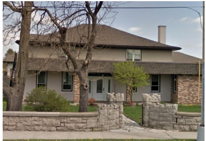
The renovated Binkley house at 500 Mohawk Road West is now St. Martin's Manor. The elegant front entrance is a replica of the original. David Lindeman photo
