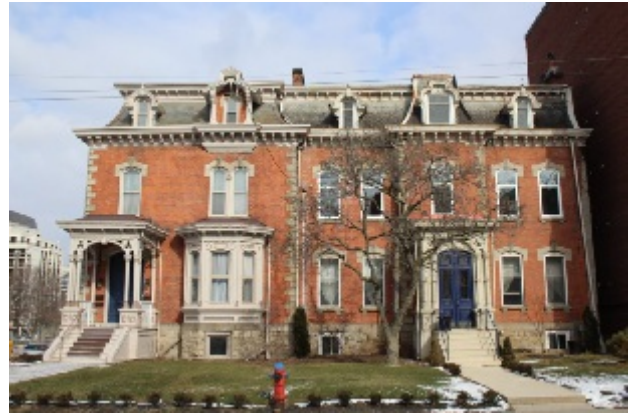
Source: the inlet on line Terrace Homes designed by James Balfour 1877, at 46 Herkimer Street, one of his 35 city building designs.
